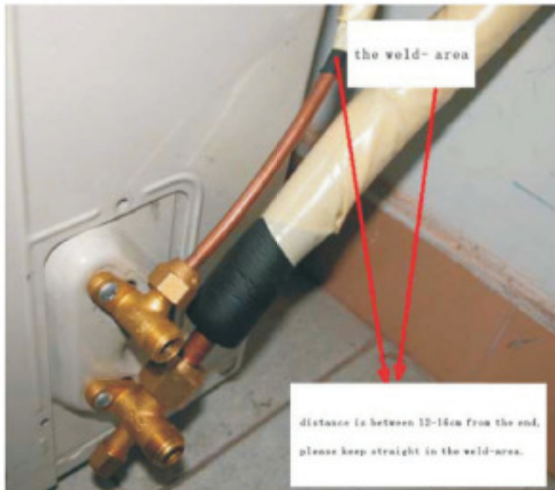
picture4 don't crinkle in the weld- area with the copper pipe and the aluminum pipe, please keep straight in the weld-area.
