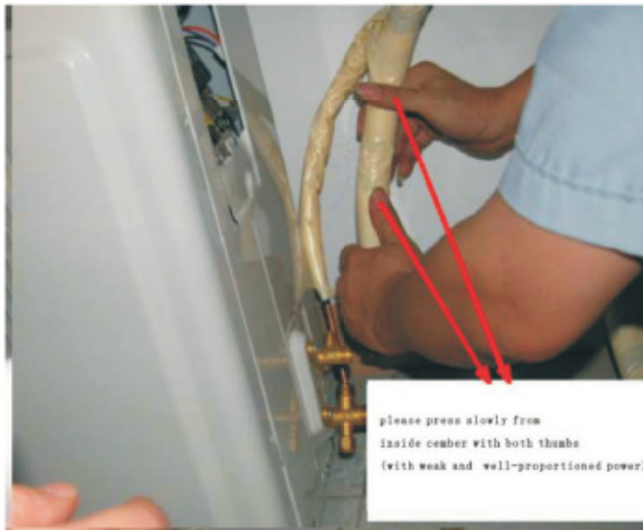
Picture 5 if could not avoid ,please press slowly from side cember by both thumbs, please press slowly from inside cember with both thumbs(with weak and well-proportioned power) .
