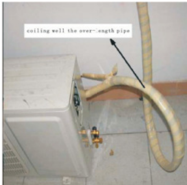
Picture 6 coiling well the over-length pipe
